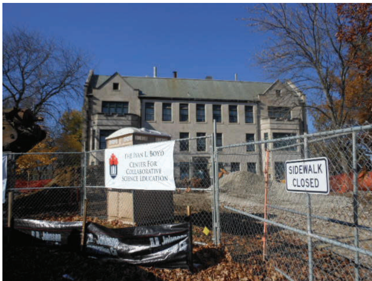
Mulvane Work in Progress
